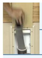
Where does the hose go? The Hide-A-Hose harnesses the suction from the power unit to retract the hose back into the PVC tubing hidden within the walls, attic, and floor joists of the home.
